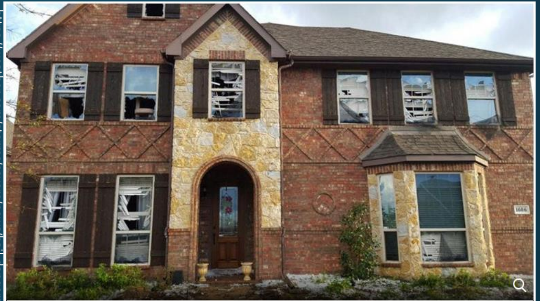
Nearly all of the windows in this Wylie, Texas, home were knocked out by a hailstorm on April 11, 2016.
